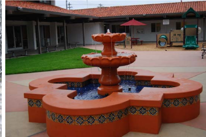
Class A – Unacceptable – Proximity to children – Needs additional barrier
