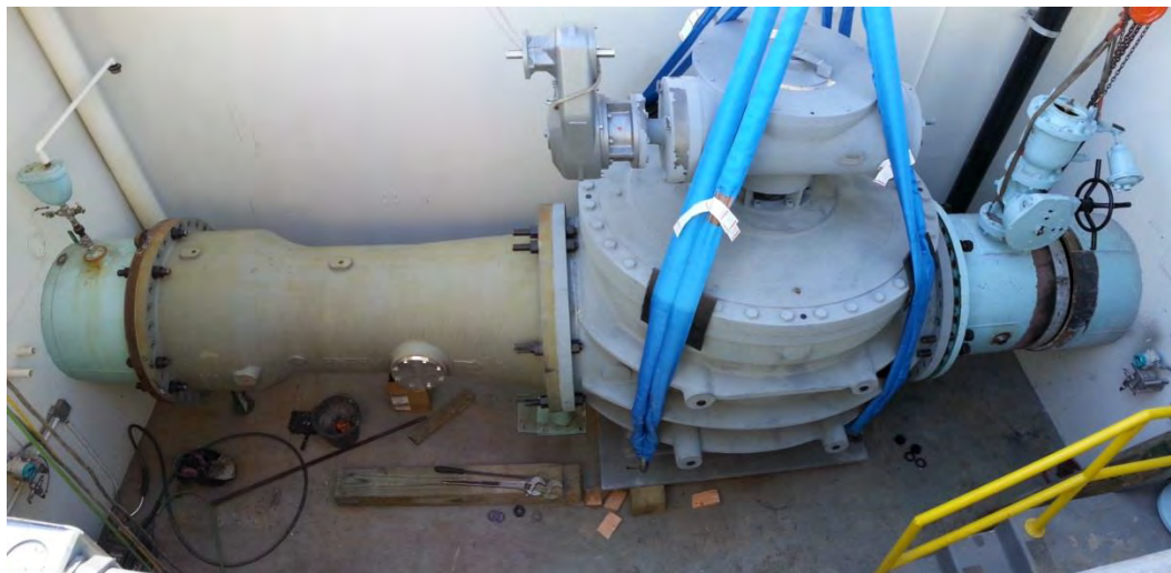
Figure 12 – San Diego 11 Meter and Control Valve Replacement
