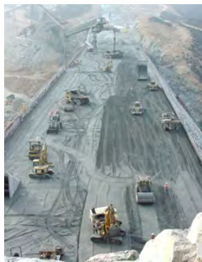
Dam construction looked like street paving.
