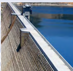
The dam has a stair-stepped appearance.
