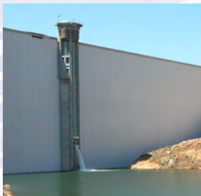
The inlet-outlet tower stands taller the dam.
